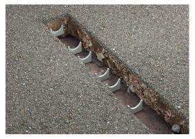
Lay the EPS supports on the bottom of the excavation site suitably compacted and leveled.
