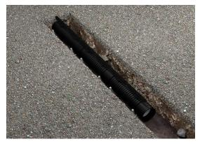
Insert the cones connecting one to the other with the special malefemale interlocking system through a rotating move on the horizontal axis and make sure they are aligned.
