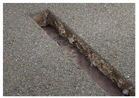
Realize the excavation according to the dimensions required in the project.
